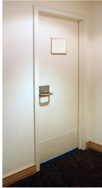
Figure 6.12: Door with undercut
