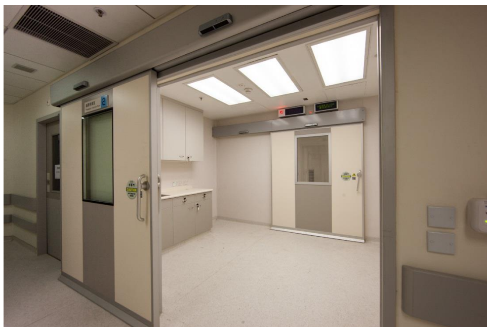
Figure 6.14: Surface mounted automatic sliding doors to Anaesthetic and Operating Rooms
