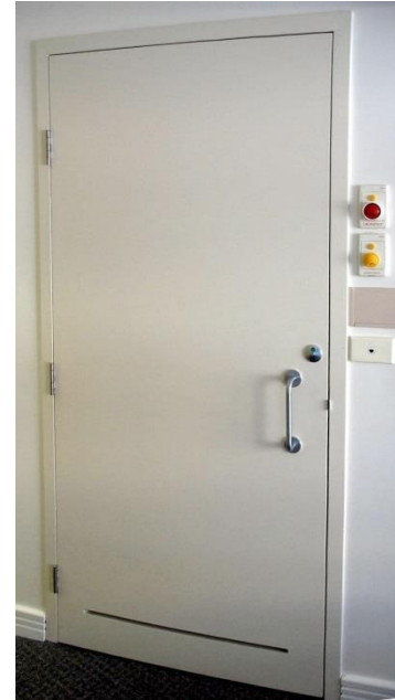
Figure 6.13: Door with slot
